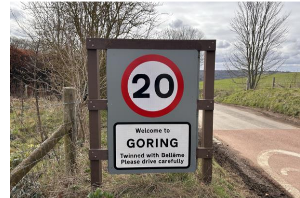
Speed calming measures can serve as gateway features as part of a Traffic in Villages approach (Goring)
