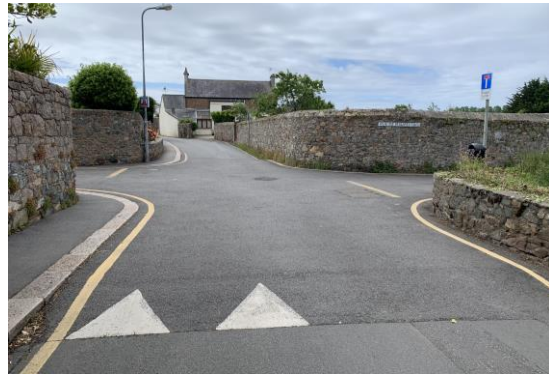
Raised table can be used on rural lane to encourage slower speeds where sightlines are poor (Jersey)
