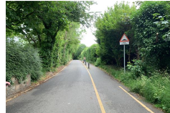
Bollards spaced intermittently along quieter rural roads can provide protected space for vulnerable users (Jersey)
